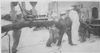
The midpoint of turnaround comes when the wharfingers fasten the hose to the deck connections of a tanker. Coordination of all factors makes fast turnaround possible.
